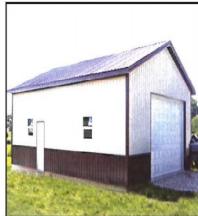
Pole Buildings and Garages
